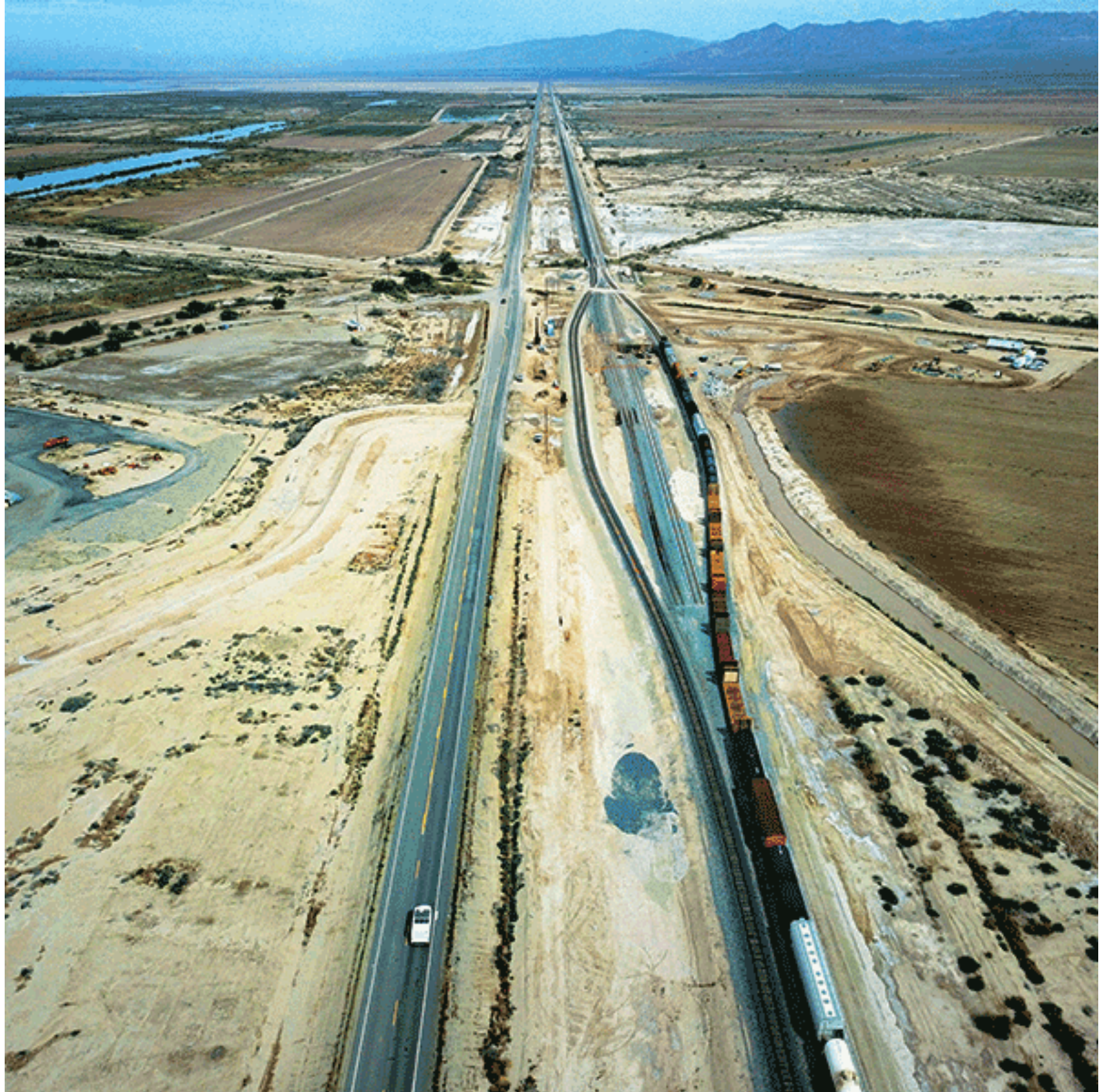
A moving mud spring developed in 2016 in Imperial County, California, that threatened railroad tracks and other local infrastructure. (David K. Lynch)
